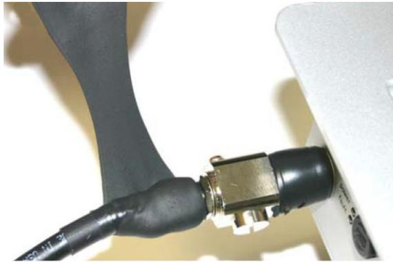
6. Wrap a layer of electrical tape (smooth side out, sticky side in) over the mastic tape.
